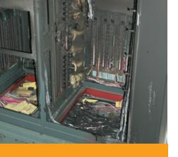
A small fire in a single cabinet, unchecked, can easily grow to consume adjacent cabinets - or even spread throughout a facility.
