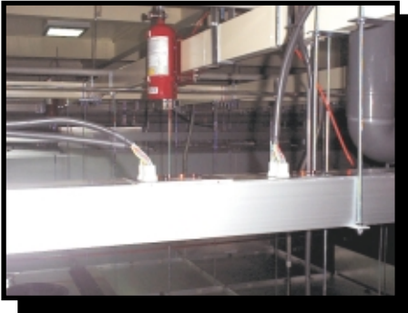
Image 1 - Elevated Cable Trays
